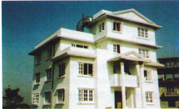
New building of WOREC
